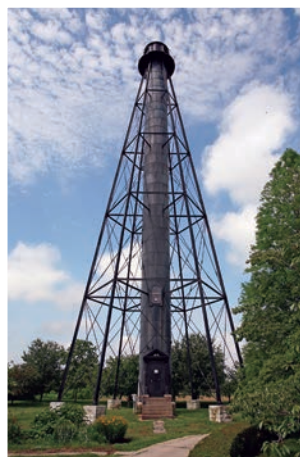
Figure 3 (above) The Liston Range Rear Light from the ground [3]
