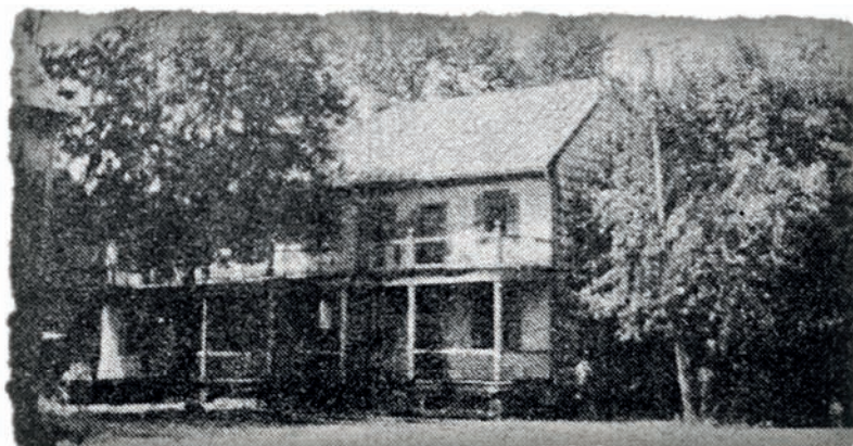
Port Penn Hotel, corner of Market and Congress Streets. Owned by: Robert Chadwick
